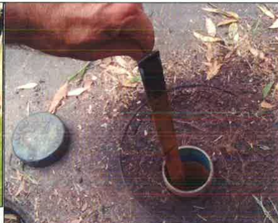
Photo 3: UST dipstick located beneath cap on concrete slab.
